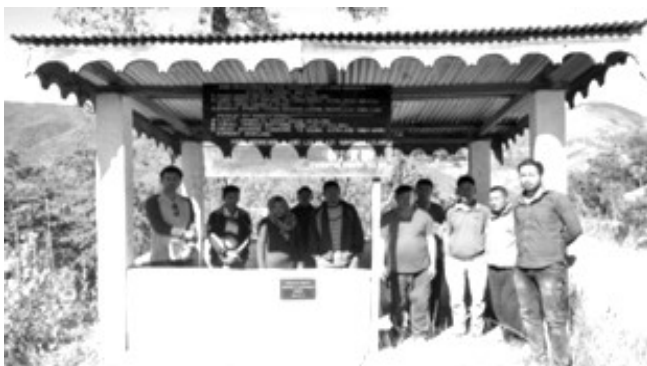
Resting Shade Construction under EPA at Tuensang Village under Tuensang district
